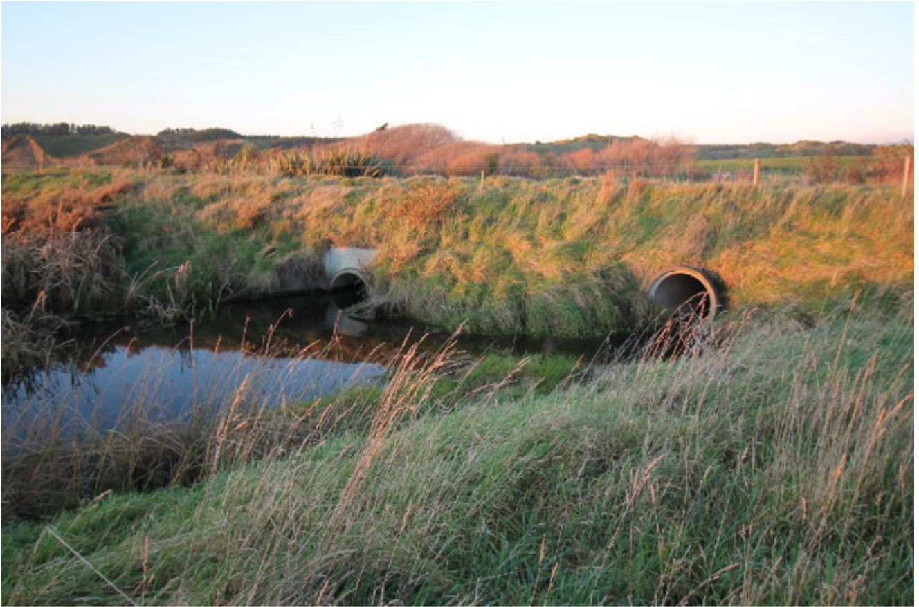
Figure A.18: Opposite view - Loop terminus with culverts exiting through to flood gates. Image Hayden Fowler 2021.
