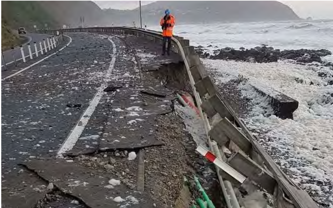
Figure 2.2 Photo taken during recent storm showing destruction of Gita Cyclone on Centennial Highway or State Highway 1 in Kāpiti region, near Pukerua Bay, 2018
