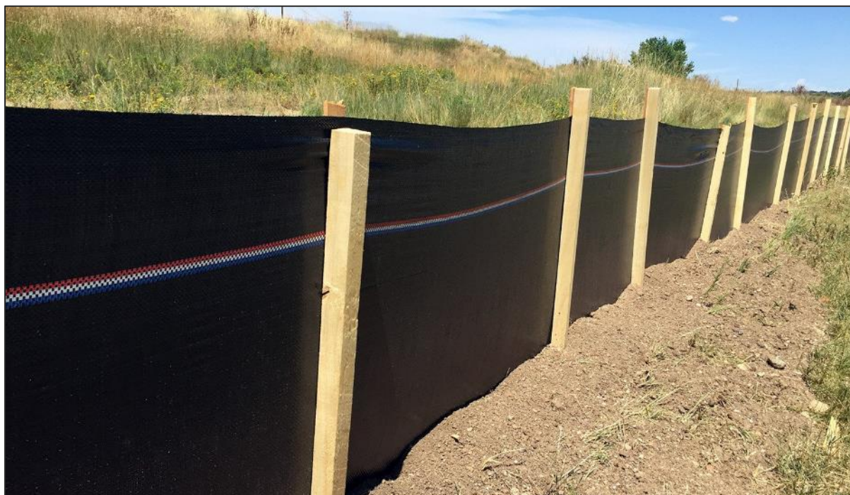
Figure 3.8: A silt fence used for erosion and sediment control
