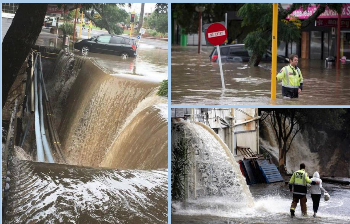
Flooding and scour damage in New Lynn during March 2017. Source: NZ Herald, Jason Valentine-Burt (left), Dean Purcell (right)
