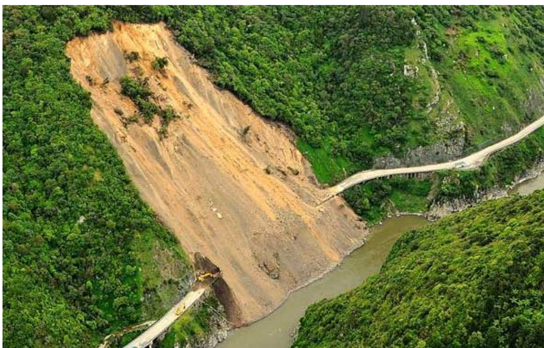
Figure 4.1: Landslide in the Manawatu Gorge (Source: NZTA)
