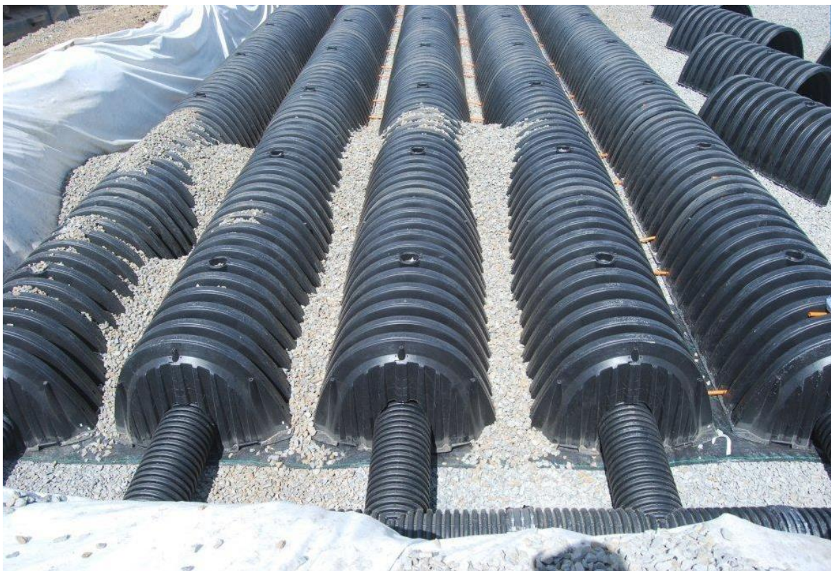
Figure 3.7: Stormwater detention and infiltration chamber system (Source: Humes, ChamberMaxx)
