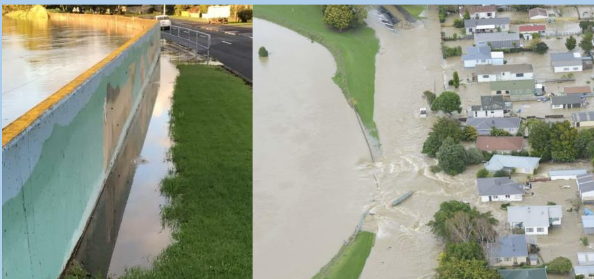
Seepage immediately in front of the floodwall at 07:04 on 6 April (left). The breached College Road floodwall at 11:00 on 6 April (right). Source for both: (Rangitāiki River Scheme Review Panel, 2017).
